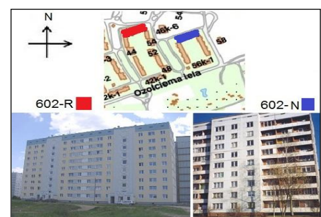
Figure 2. 602.series MAB photo and schematic location (renovated: 602-R; not renovated: 602-N)
