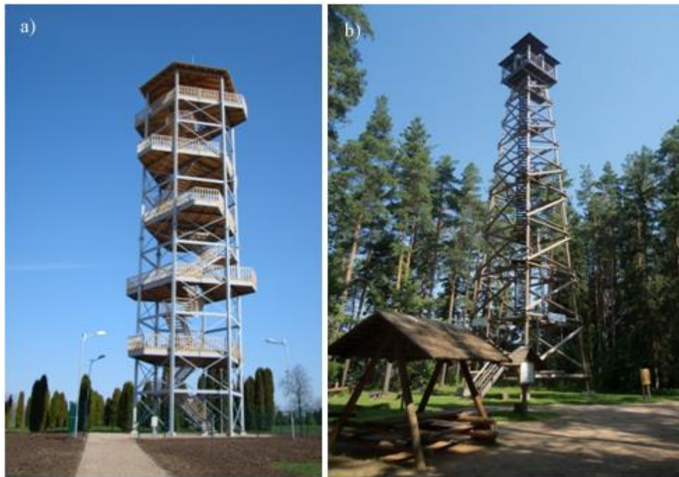
Figure 2. a) An example of the steel observation tower (in Kalsnava); b) An example of the timber observation tower in the region of Latgale (Priedaine)
