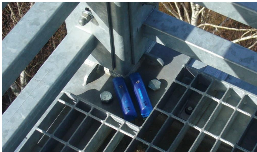
Figure 3.1. Arrangement of accelerometers on the tower in Dzintari
