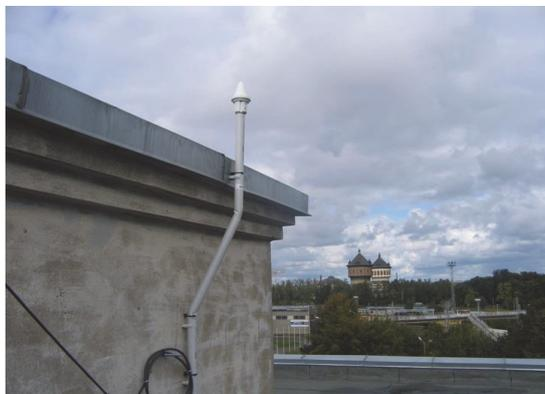
**Fig. 3.3.** Receiving antenna of GPS signal retranslation system at RTU TET department.
