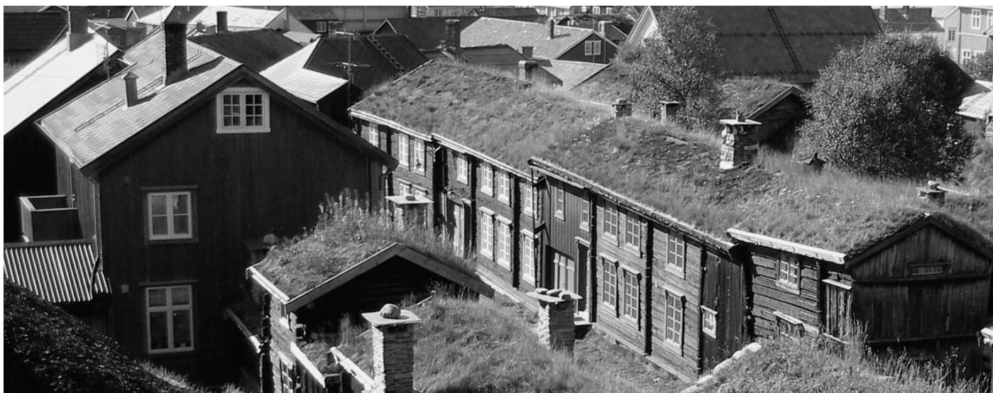
Fig. 4. The dwelling-house (Sleggveien 3) in the left corner of the picture was considered as of poor quality and was decided by the National Directorate for Cultural Heritage to be demolished in the 1950-ties as it ruined the “true image of Røros” by creating the dissonance to its surroundings. (Photo taken by Giedrė Jarulaitienė, 2008).
