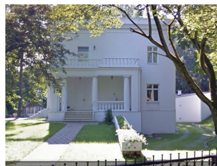
Bruža house, 2018 [Photo: B.Vērpe].
