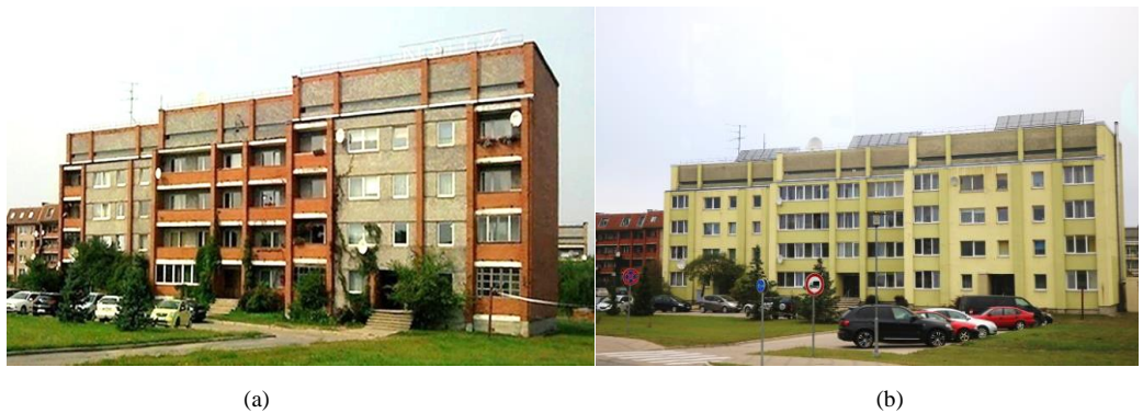
Fig. 1. Building 3: a) before renovation; b) after renovation.
