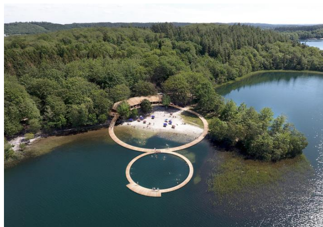
Figure 70. Eastern and Western Bathing Resort, Sweco Architects, Denmark [Photo by Sweco Denmark, Annex 7].
