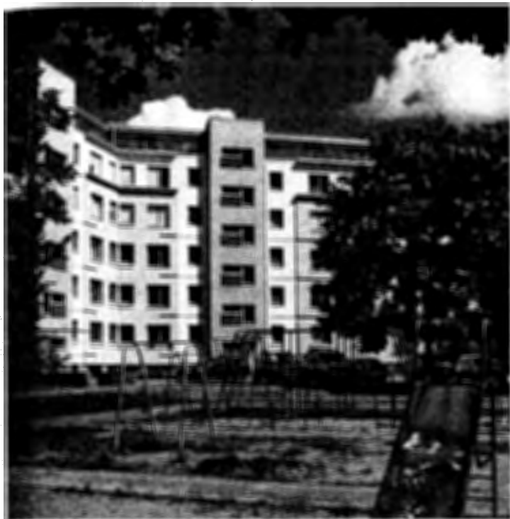
Fig. 4. The old playground next to the new building. (Photo by Edgars Suvorovs)
