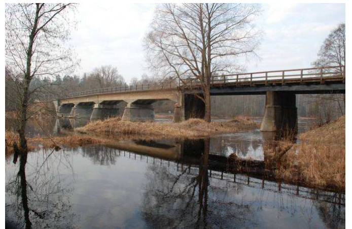
Fig.2. The bridge over Gauja river near city of Stenci, built in 1909
