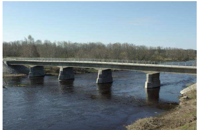
Fig.1. The bridge over Salaca river, built in 1908
