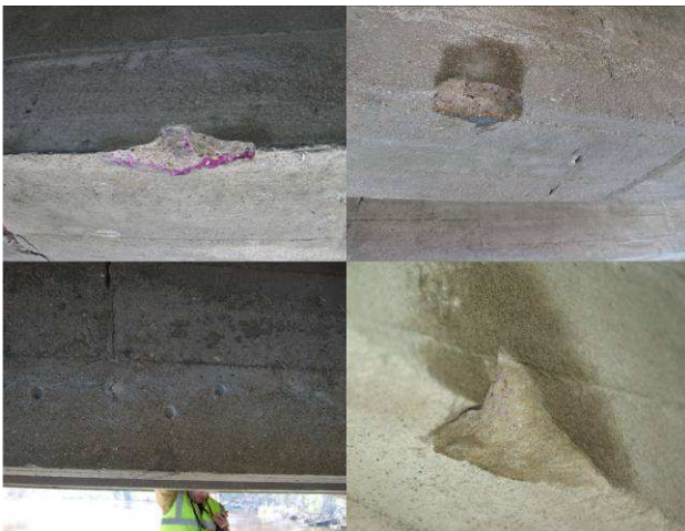
Fig. 12. Determination of the depth of carbonation of the concrete
