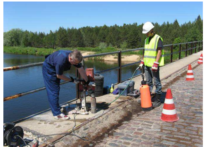
Fig. 13. Concrete core drilling
