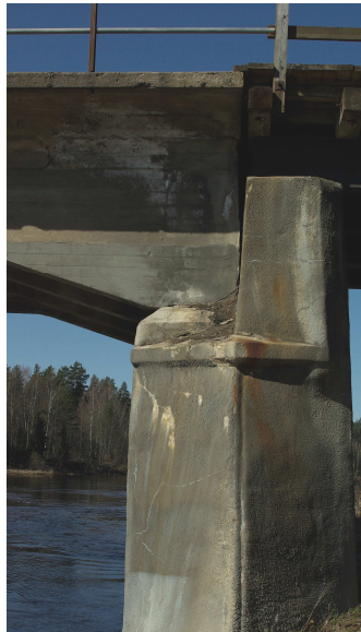
Fig.7. Repaired pier in 2008
