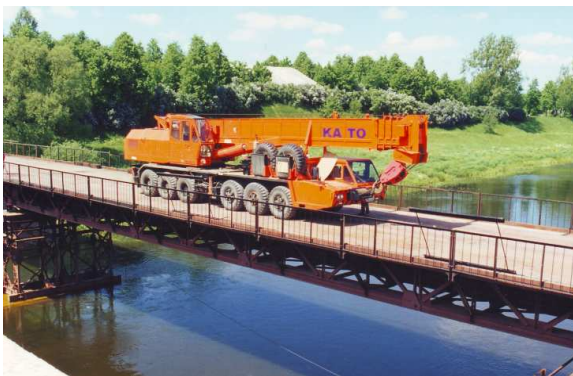
Fig. 4. Crane as an example of the heavy weight (60 t) traffic load
