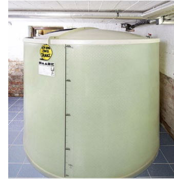
Oil tank made for GRP www.haasetankhamburg.de
