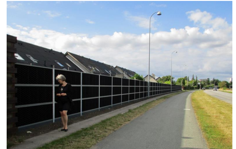
Sustainable, efficient noise barrier
