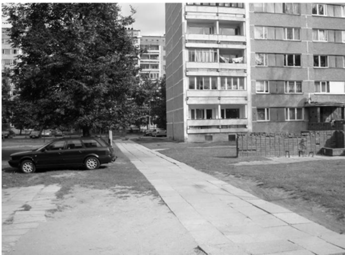
Fig. 4. Disorganized functional zones of a courtyard in Jelgava (Photo by Una Īle, 2009)
