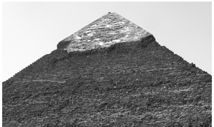
Fig.6. The Pyramid of Khafre at Giza with the remains of casing from Tura-Maasara quarry
