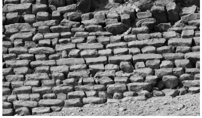
Fig. 5. Building blocks used in the fourth step of the construction of the Step Pyramid (southern façade)
