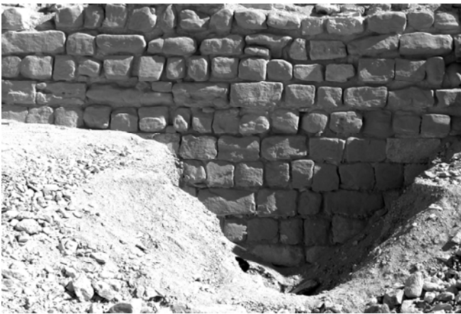
Fig. 4. Building blocks used at the base or "0" step at the western façade of the Step Pyramid
