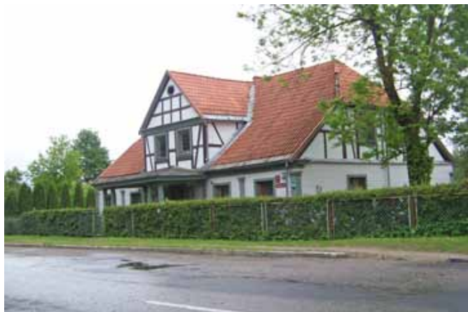
Fig. 3. The restored residential house at Dambja iela 17.
