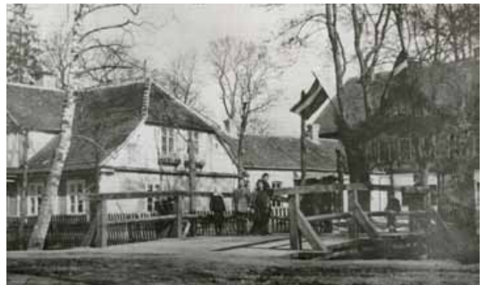
Fig. 1. The historical building along Duke Jacob's Canal (the 30s of the 20th century).
