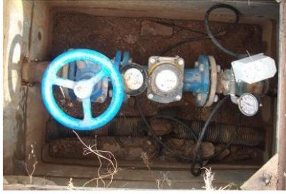
Fig. 4.1. Water supply control unit
