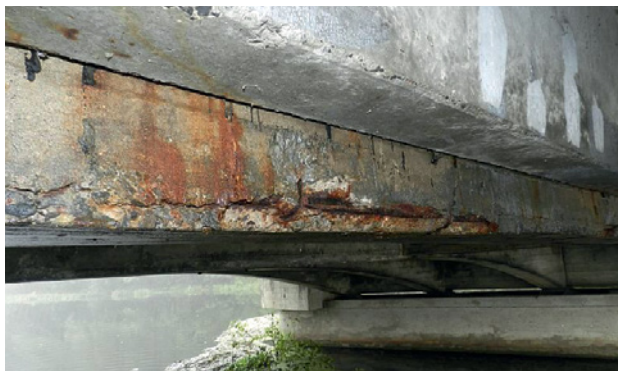
Figure 3. The initially outermost Reinforced Concrete girder covered by the added I-girder (photo A. Madaj)
