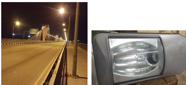
Fig. 3. “Dienvidu tilts” bridge and ONYX2 luminary.
