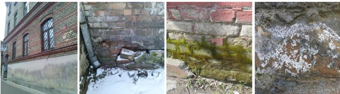
Fig. 2.2. Damages caused by moisture in masonry of historic buildings.
