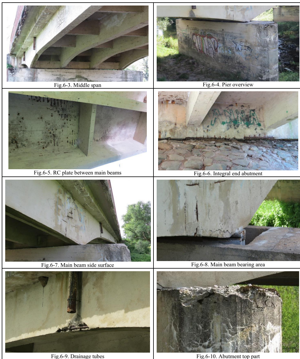
Figure 6. Overview of bridge main defects
