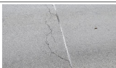
Fig.6-2. Saw cut in asphalt pavement
