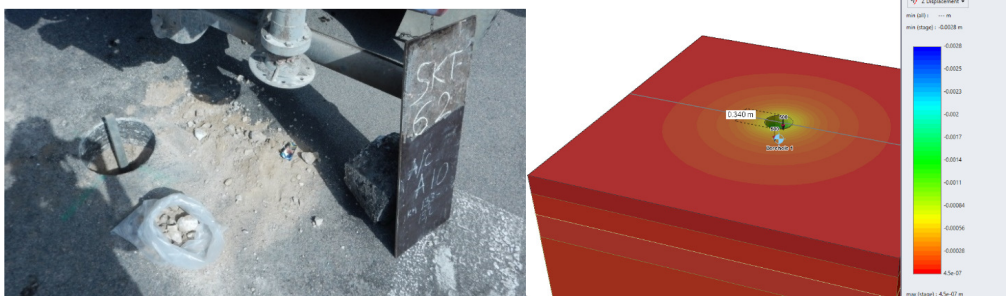
Figure 10. Geotechnical research trial test pit at section 16.4km
