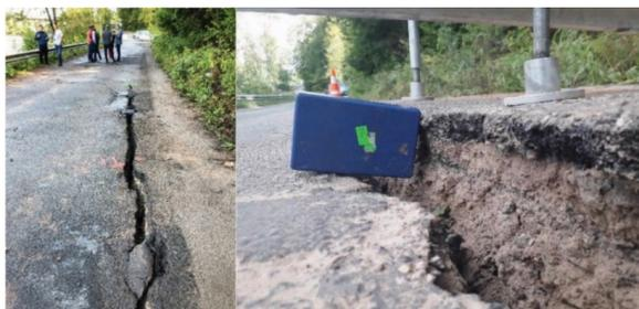
Fig. 3.2. Deformations of *Peldu* street road structure.
